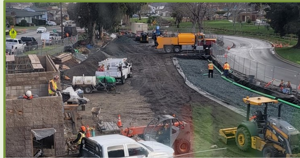
Parking Lot Sidewalk and Curbs
