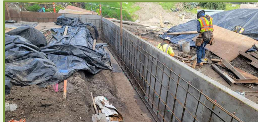
Kid's Play Yard Wall Foundation
