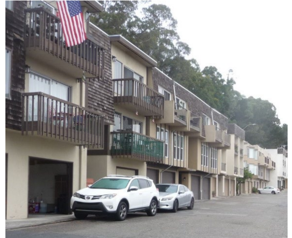
These cars are not parked legally, as they block the garage entrance. Parking is not permitted on this street as it was not built to a width to accommodate parking on the street.
