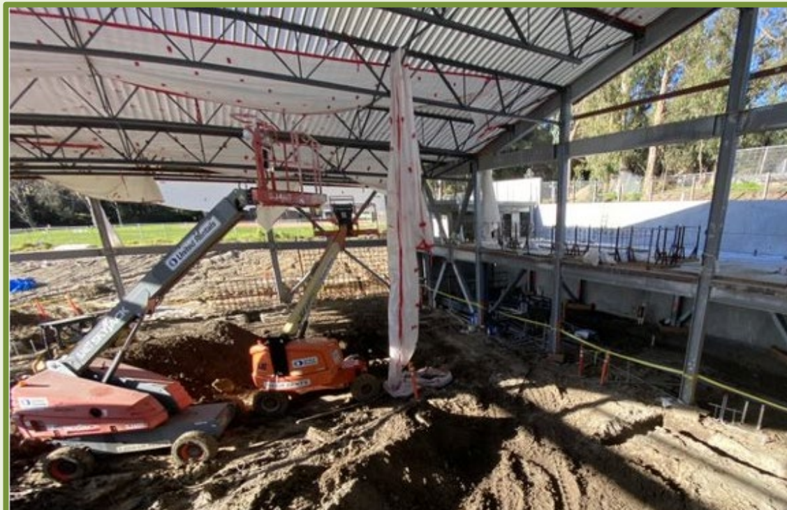
ROOF TRUSS RUST PROOFING - STARTED
