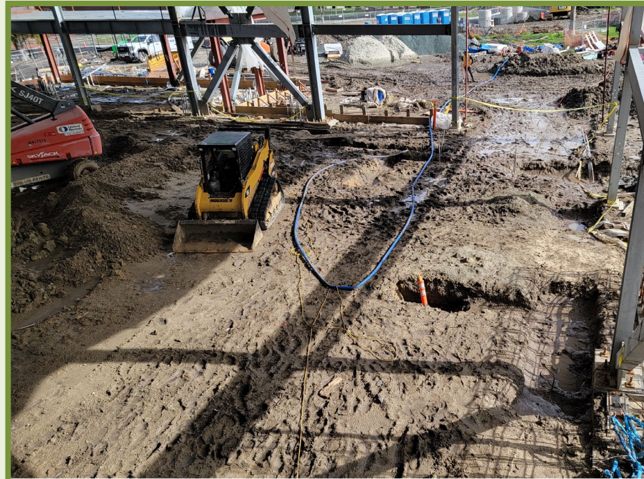
INDOOR POOL EXCAVATION PREP
