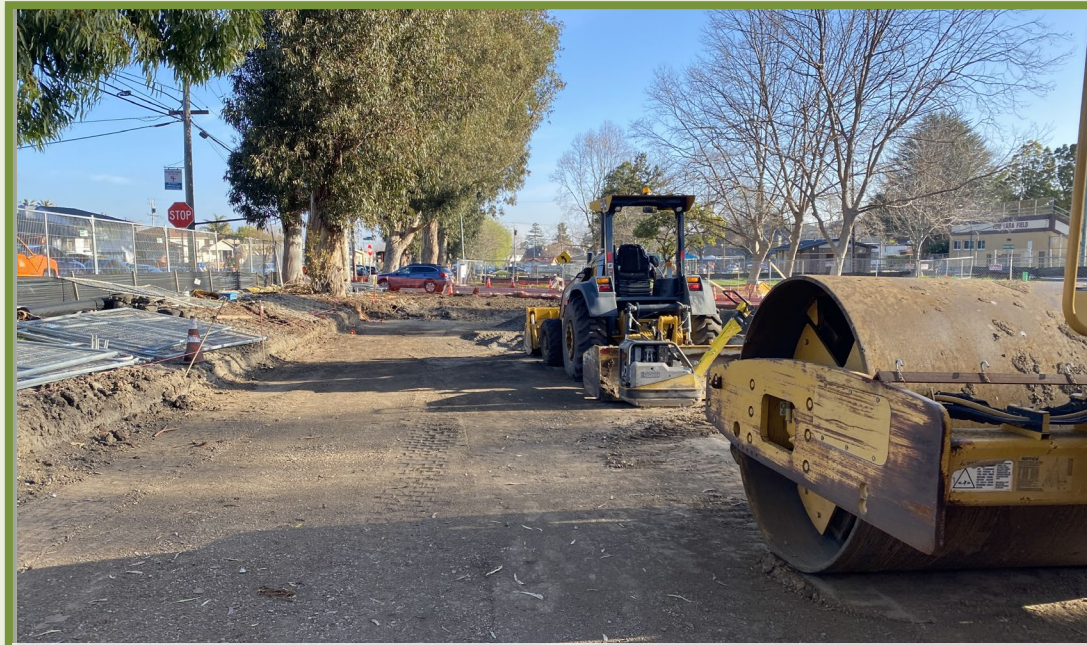
STARTED PARKING LOT GRADING
