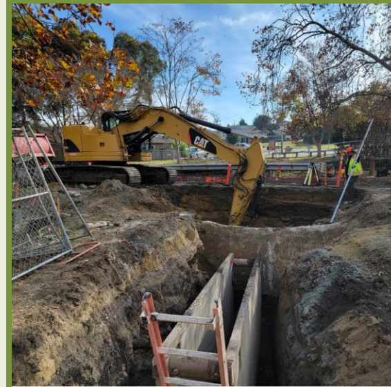
SEWER LINE INSTALLATION
