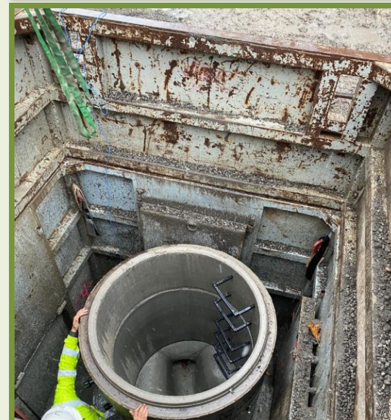
SEWER MANHOLE INSTALLATION
