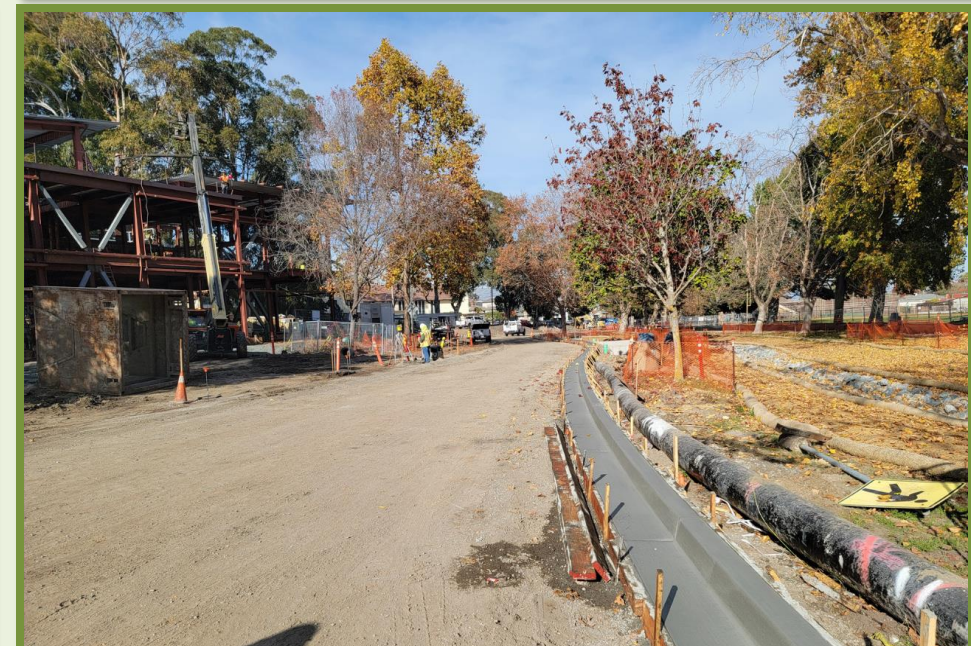
NEW CURB & GUTTER
