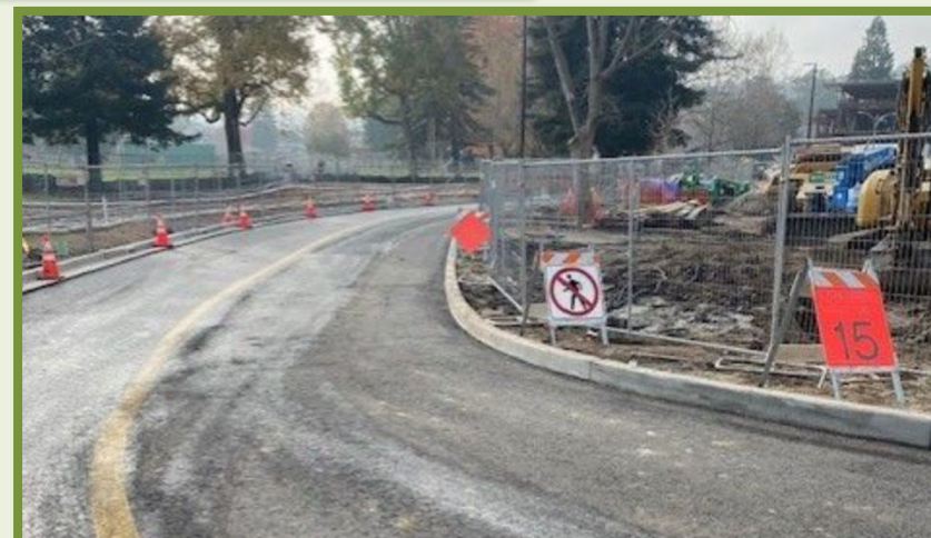
ENTRANCE TO CITY PARK WAY
