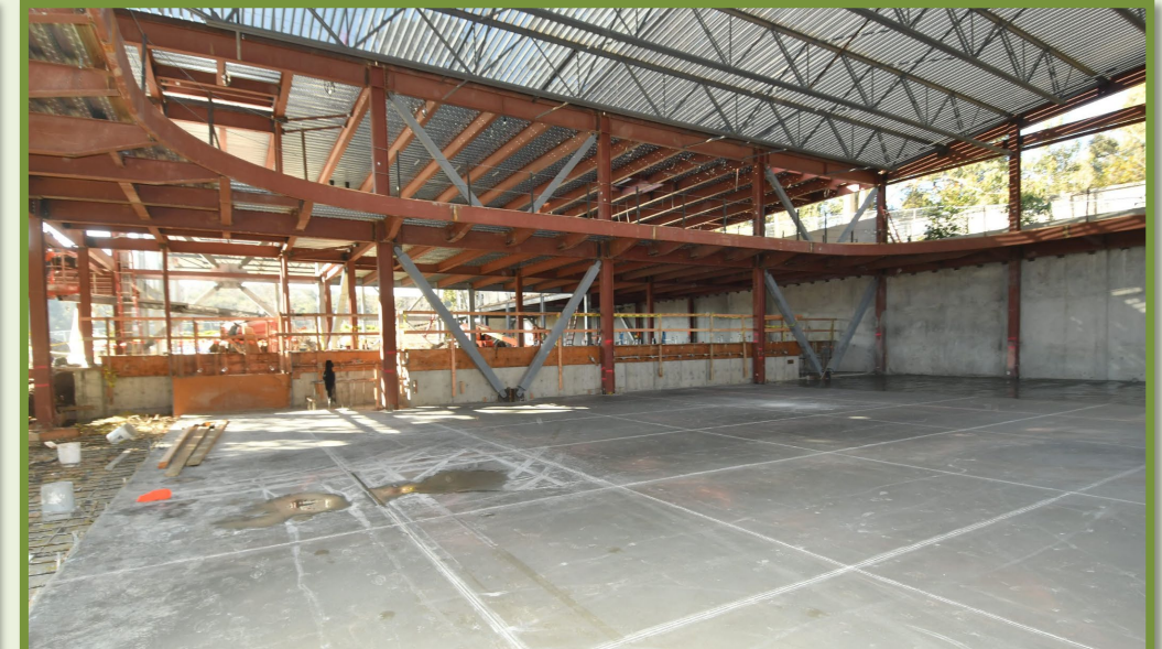
CONCRETE SLAB - GYMNASIUM
