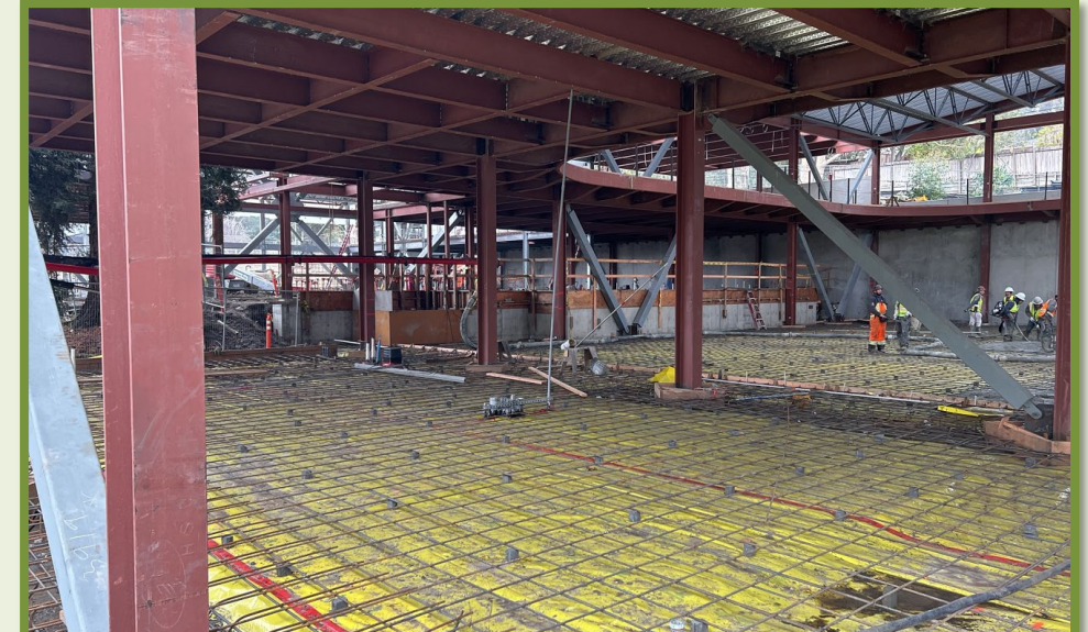
FLOOR REBAR - GYMNASIUM
