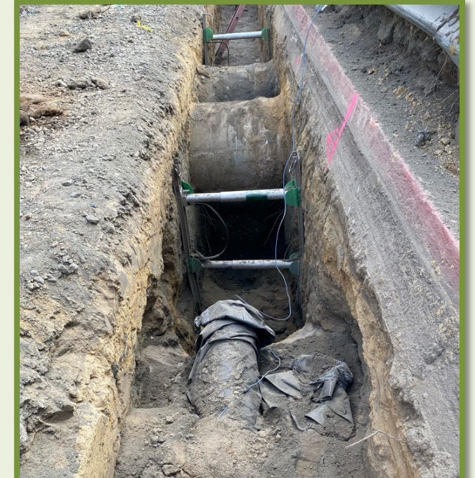
NEW WATER LINE GOING UNDER EXISTING STORM LINES
