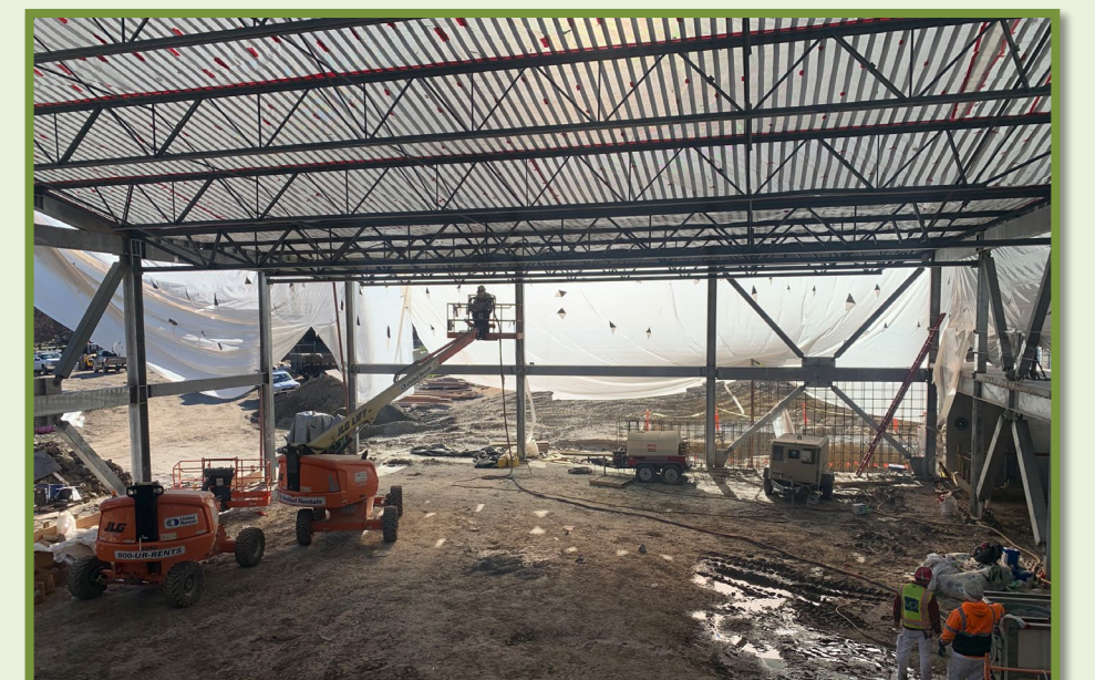
ROOF TRUSSES - NATATORIUM
