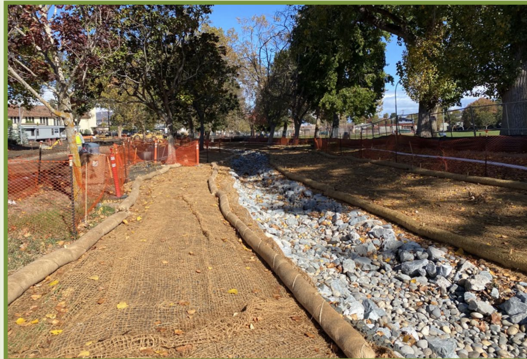
CREEK REALIGNMENT AT THE OUTFALL
