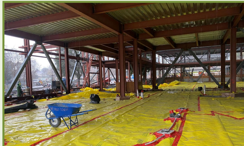
FIRST FLOOR VAPOR BARRIER - CLASSROOMS
