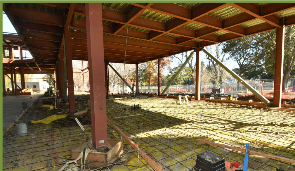
REBAR - LOBBY & SHARED OFFICE ROOMS
