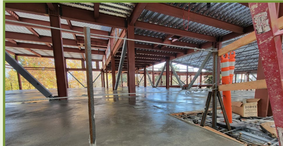
TOPPING SLAB – 2ND FLOOR COMMUNITY HALL
