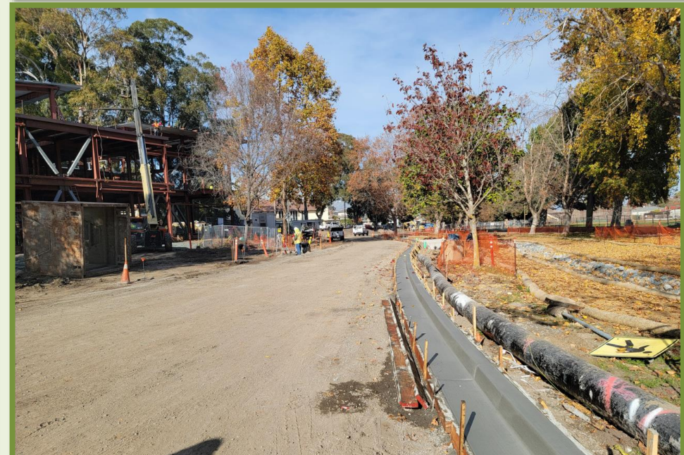
NEW CURB & GUTTER
