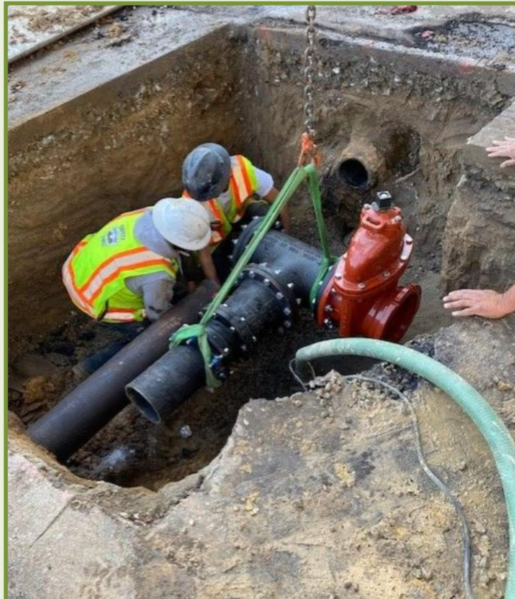
WATER TIE-IN BY DESOTO ROAD (REMOVED TEMPORARY WATER BYPASS)
