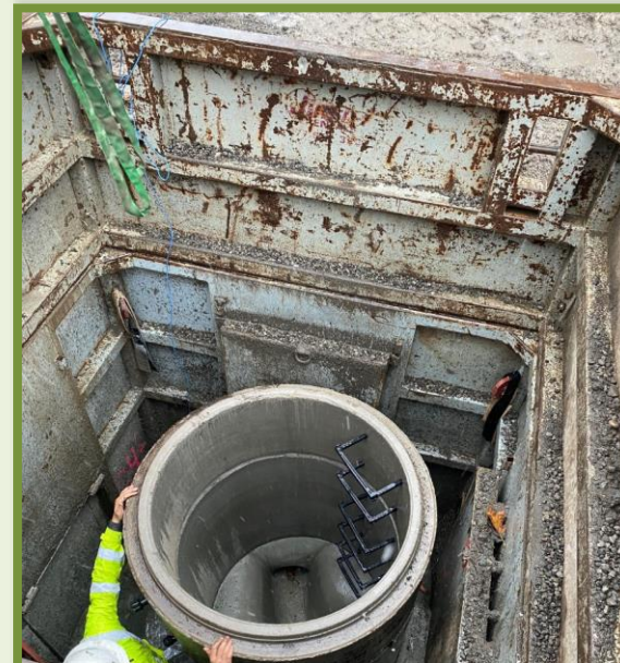
SEWER MANHOLE INSTALLATION
