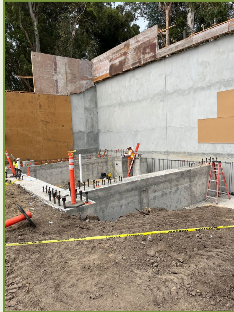
STEEL ERECTIONS PREP WORK
