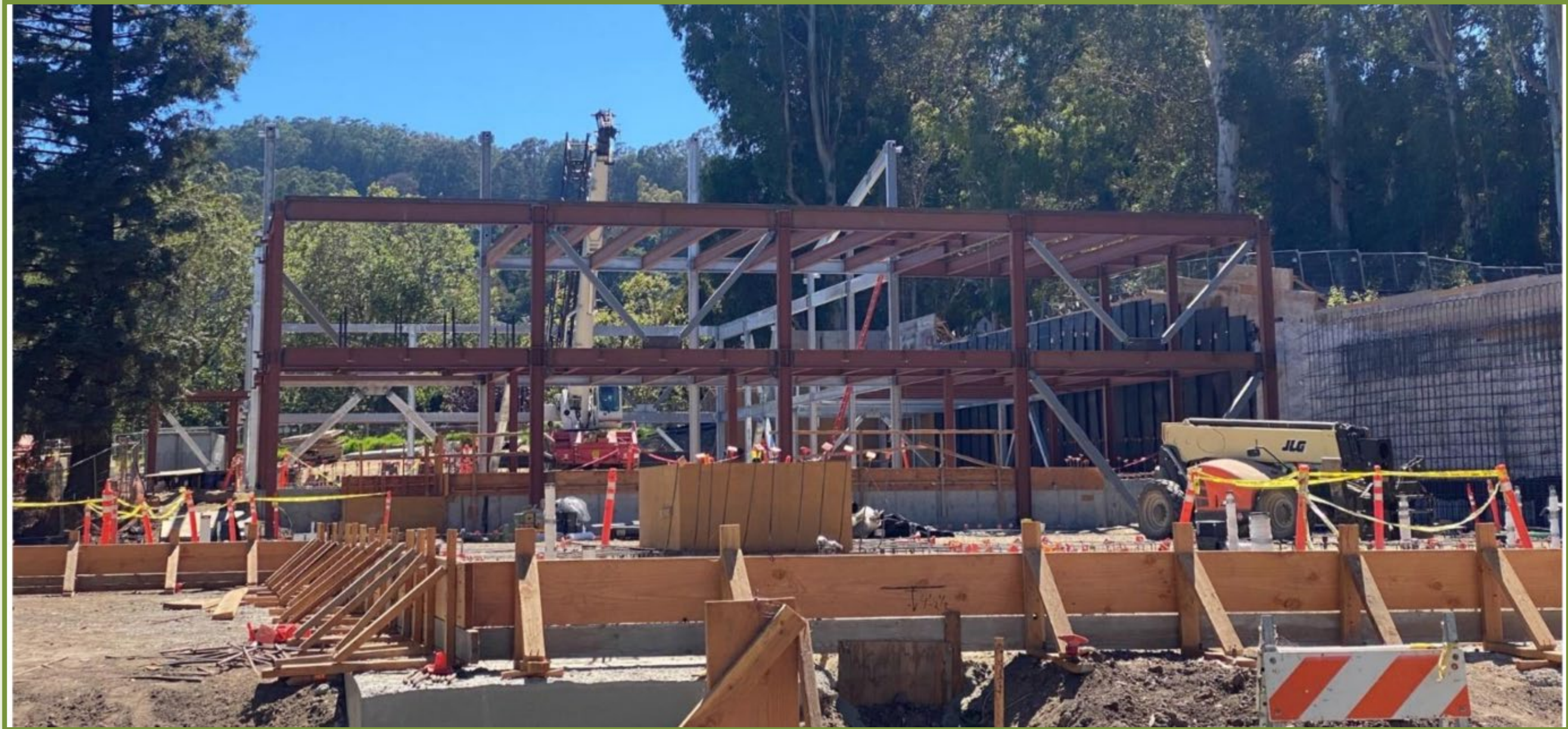
Natatorium Steel Erection Progress
