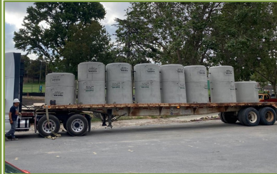
SEWER PIPE INSTALLATION PROGRESS
