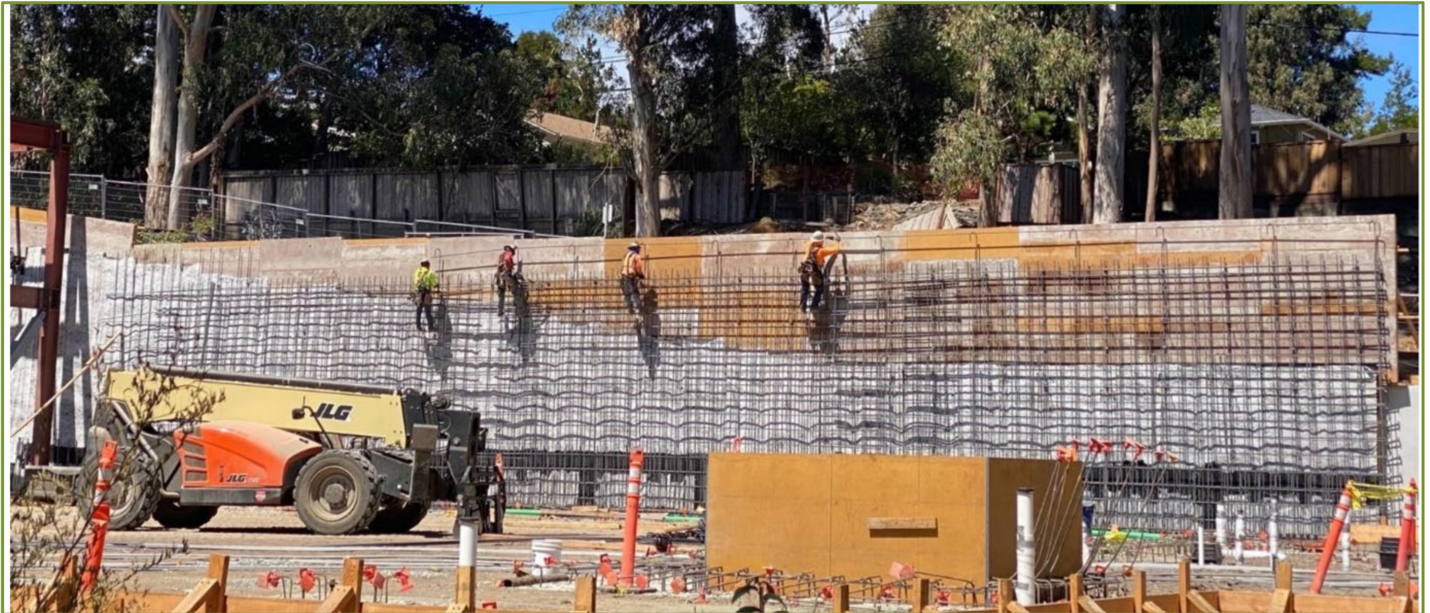
BUILDING LINE "A" WALL (Crystal Spring next to the Shoring Wall)
