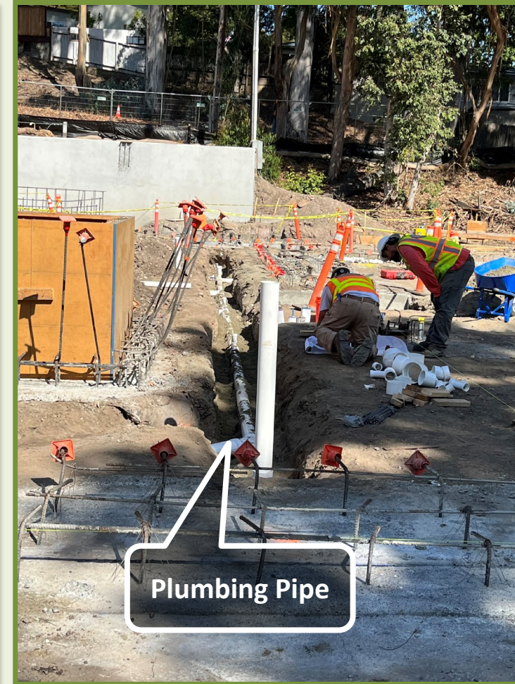
Underground related work (Plumbing and Electrical)
