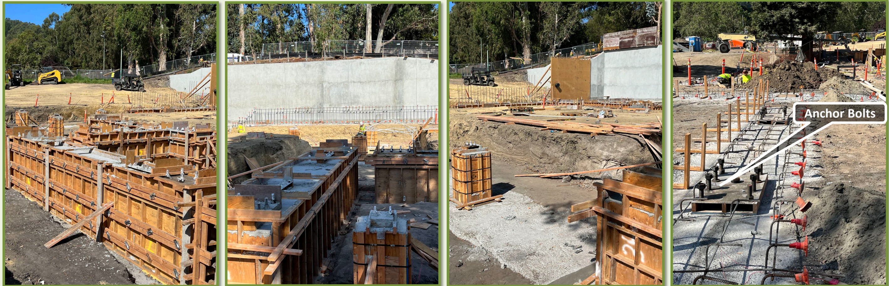
July 16, 2022 – Foundation Stem Wall / Anchor Bolts
