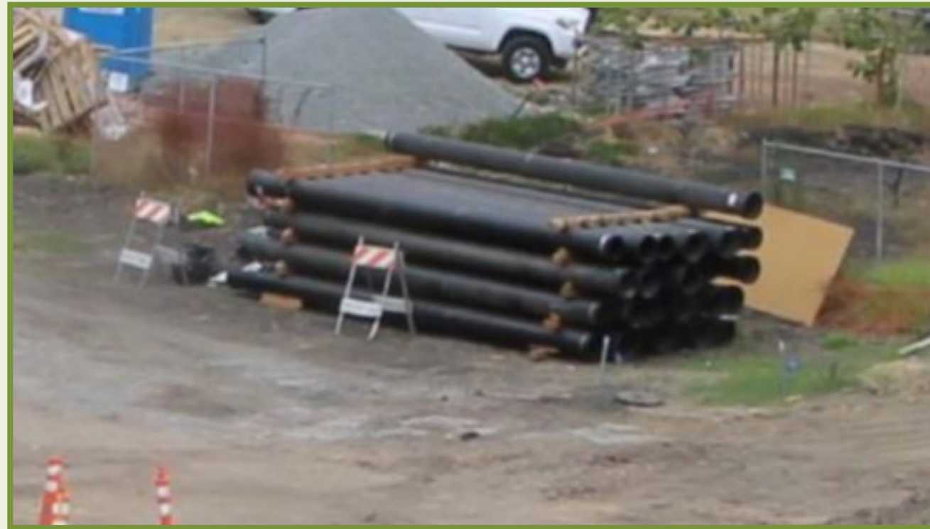
DUCTILE IRON PIPE DELIVERY Water Line Trenching – Crystal Spring
