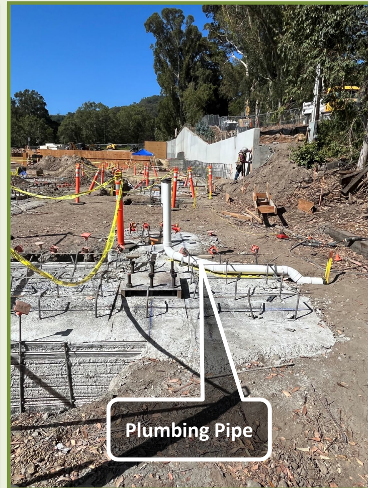
Underground related work (Plumbing and Electrical)
