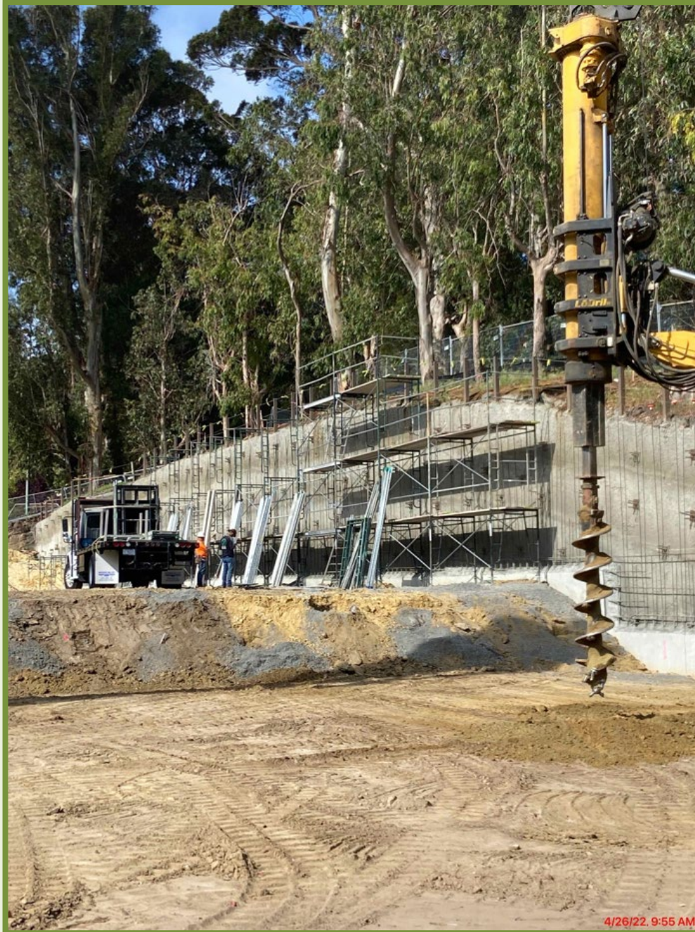
RETAINING WALL SURFACE AND GEOPIER
