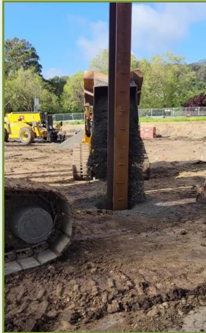
GEOPIER RIG SETTING THE RAMMED AGGREGATE
