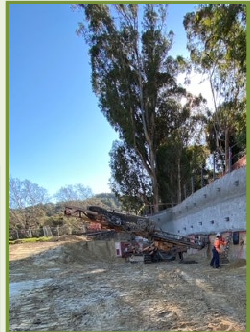
DRILLING & SETTING NAILS
