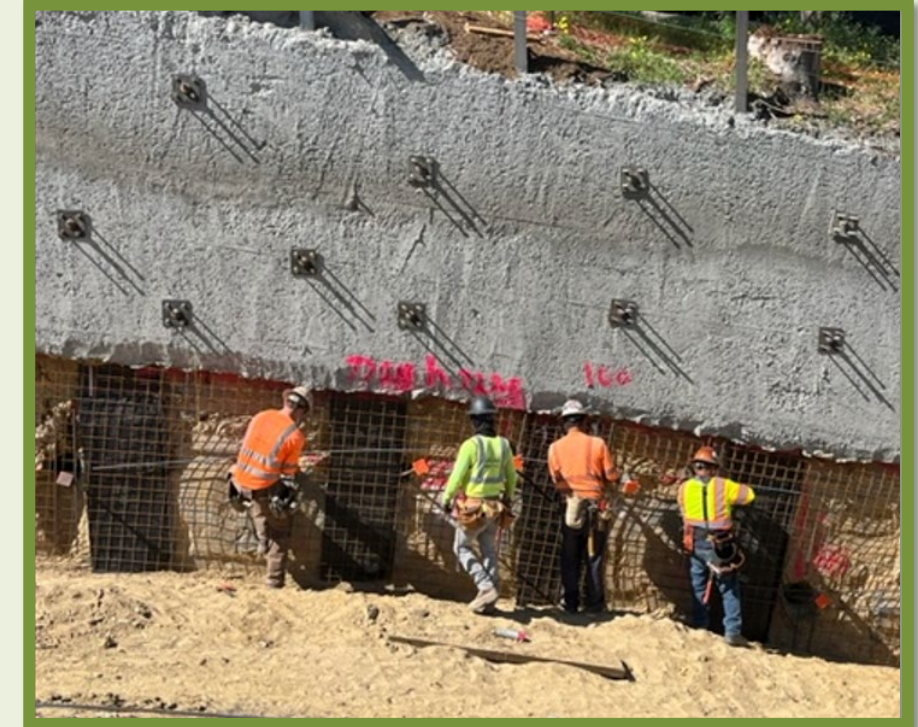
3 - GROUT, TESTING AND SHOTCRETE PREP
