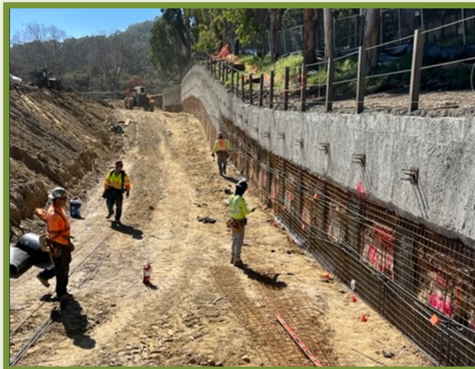
GRADING FOR NEXT LAYER
