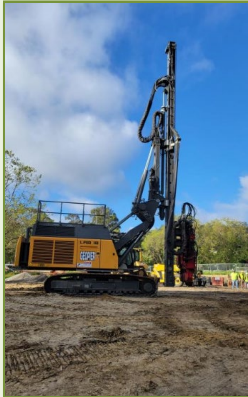
GEOPIER RIG SETTING THE RAMMED AGGREGATE
