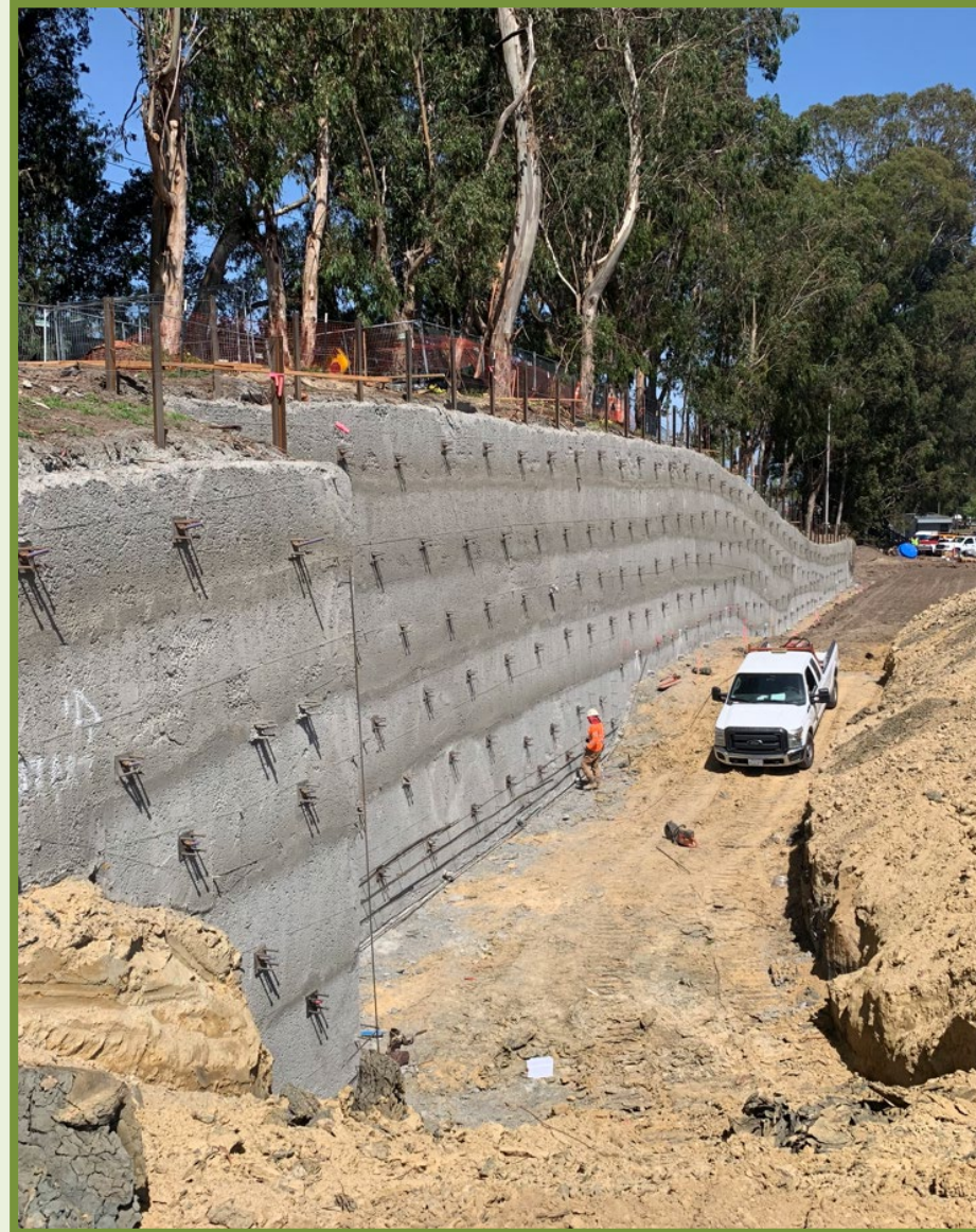
5 - COMPLETED SOIL NAIL WALL (RETAINING WALL)
