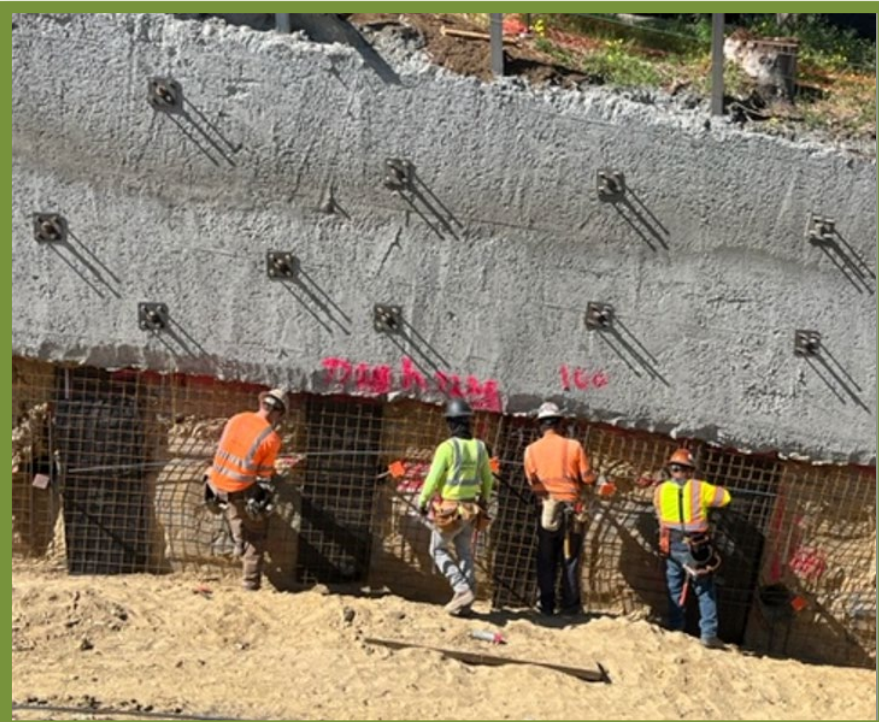
GROUT, TESTING AND SHOTCRETE PREP
