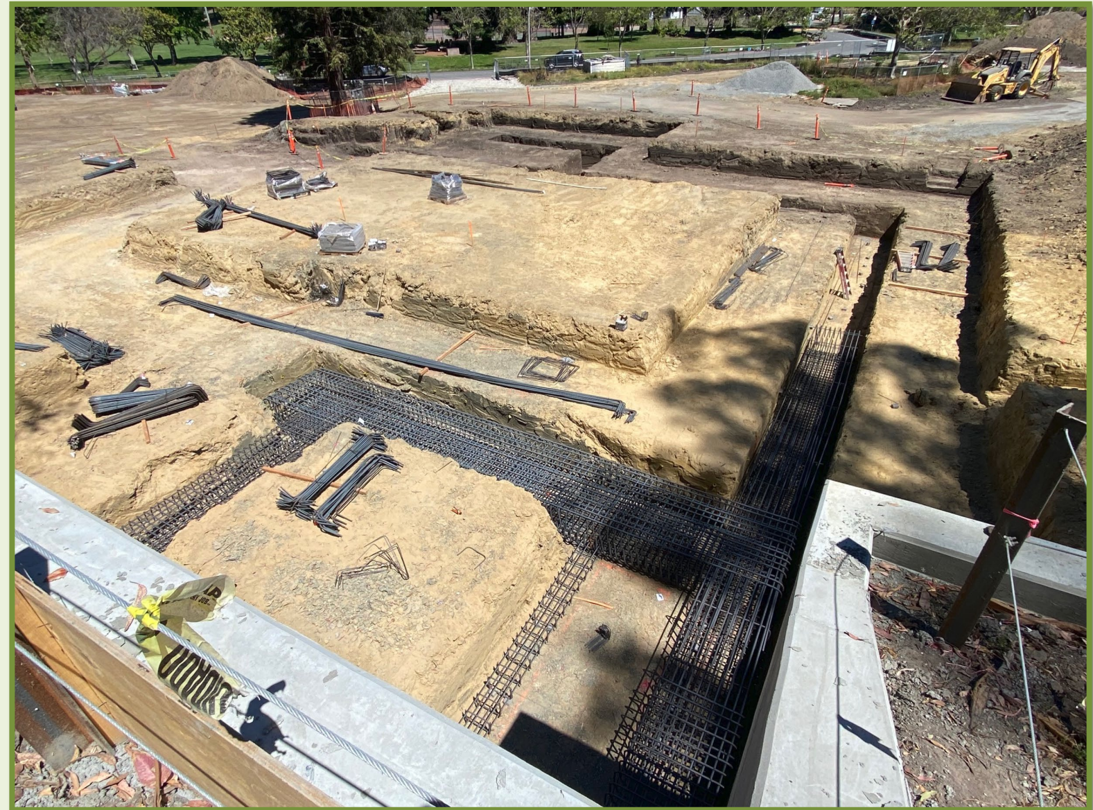
BUILDING FOUNDATION EXCAVATIONS AND REINFORCING BARS
