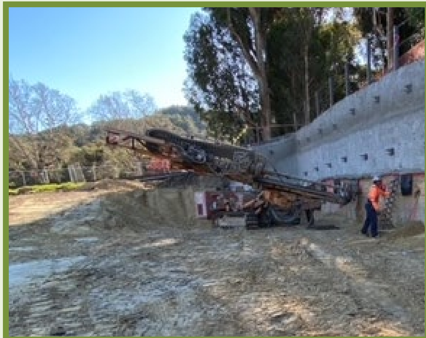
2 - DRILLING & SETTING NAILS
