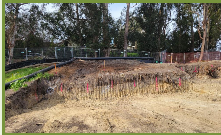
1 - CUT SLOPE, MARKED FOR SOIL NAIL DRILLING & SETTING
