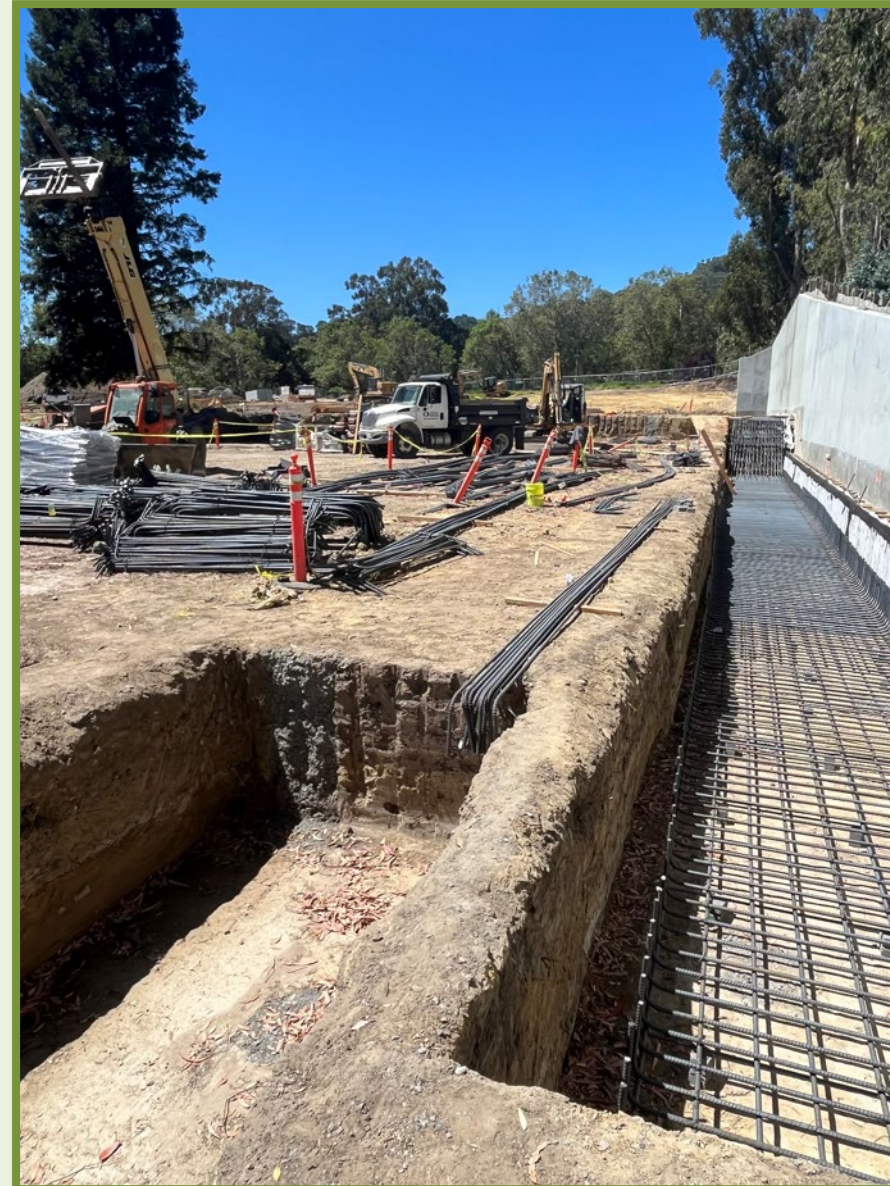
BUILDING FOUNDATION EXCAVATIONS AND REINFORCING BARS
