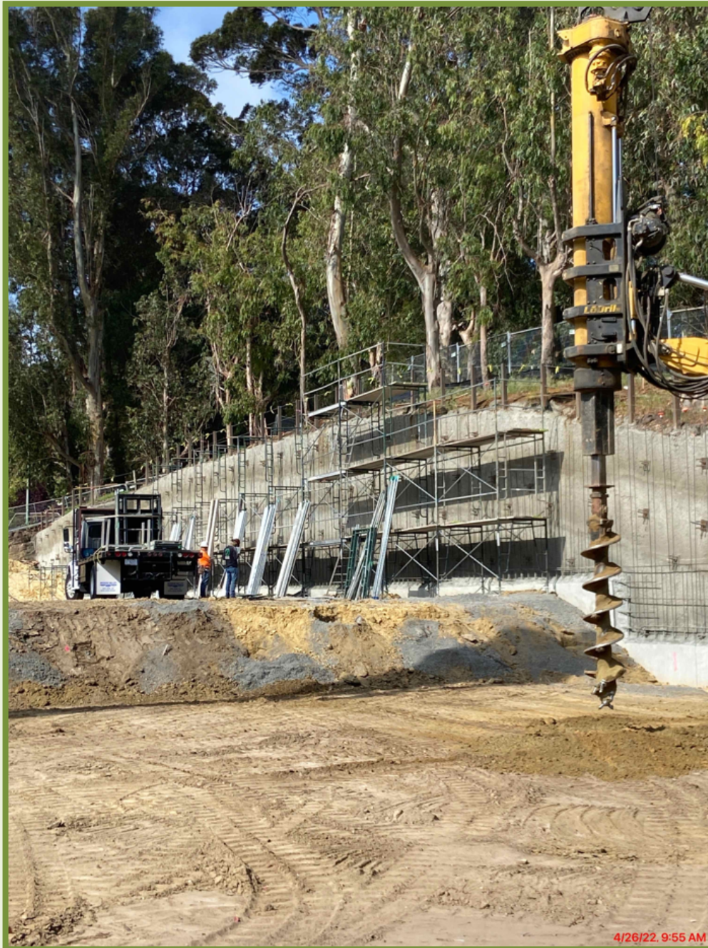
RETAINING WALL SURFACE AND GEOPIER
