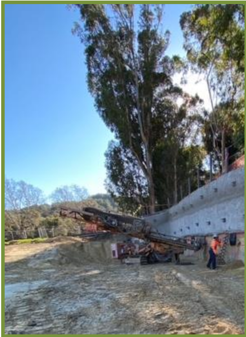
DRILLING & SETTING NAILS
