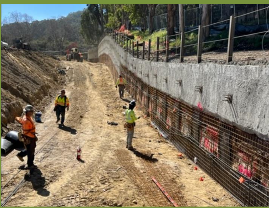
GRADING FOR NEXT LAYER
