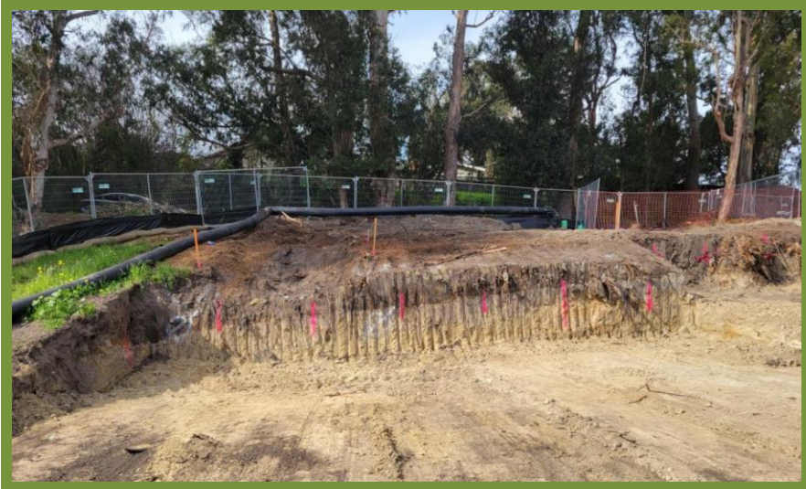
CUT SLOPE, MARKED FOR SOIL NAIL DRILLING & SETTING
