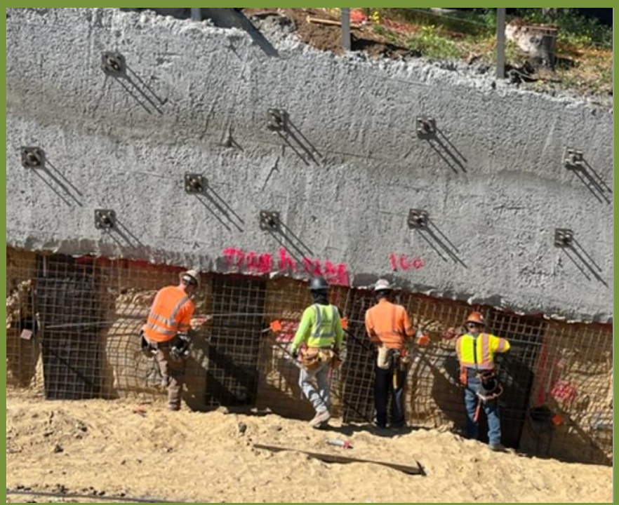
GROUT, TESTING AND SHOTCRETE PREP
