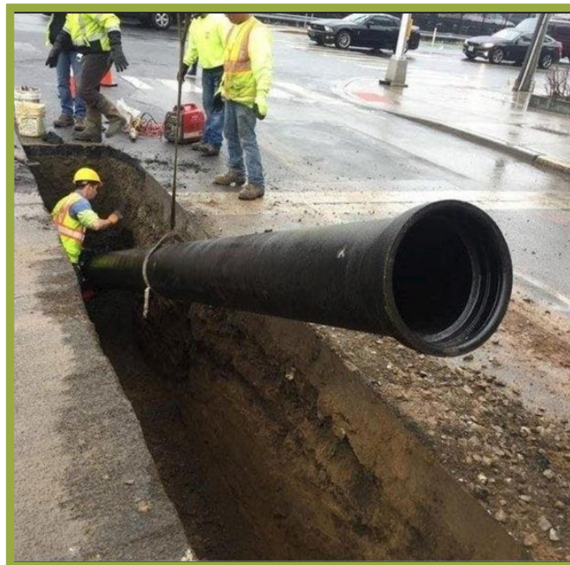
New Water Pipes
