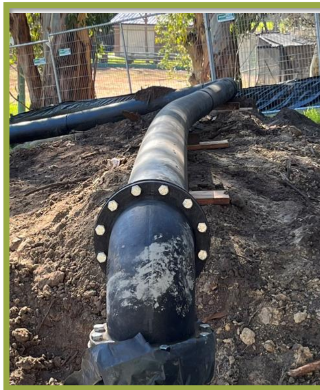
TEMPORARY WATER LINE BYPASS
