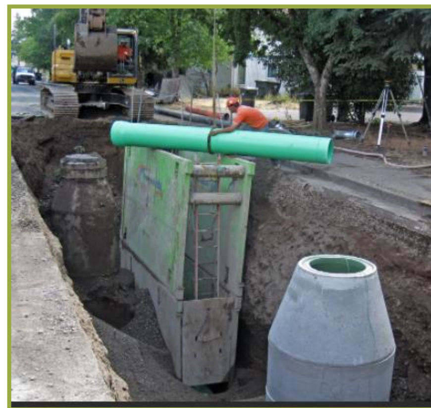
New Sewer Pipes
