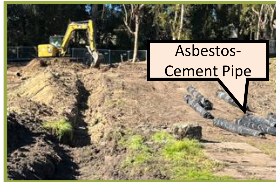
OLD WATER LINE REMOVAL
