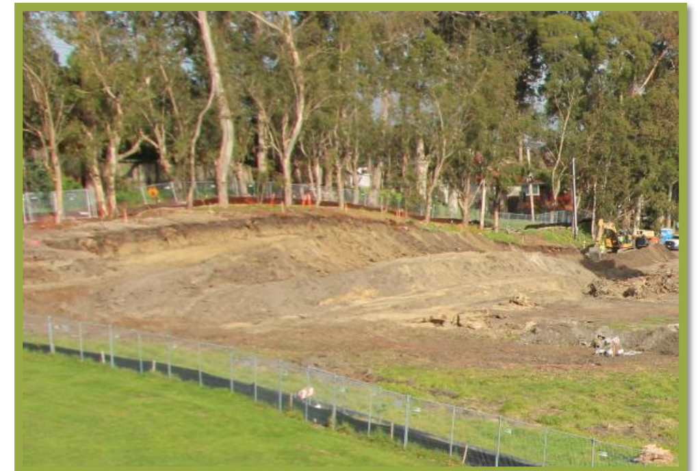
RETAINING WALL WORK
