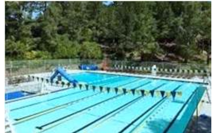
Highlands Recreation District – 6 Lanes
