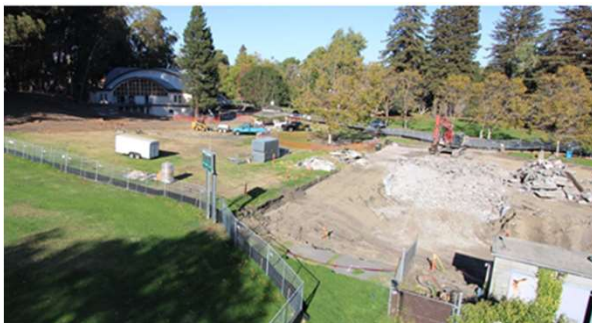
Gym Building Demo
