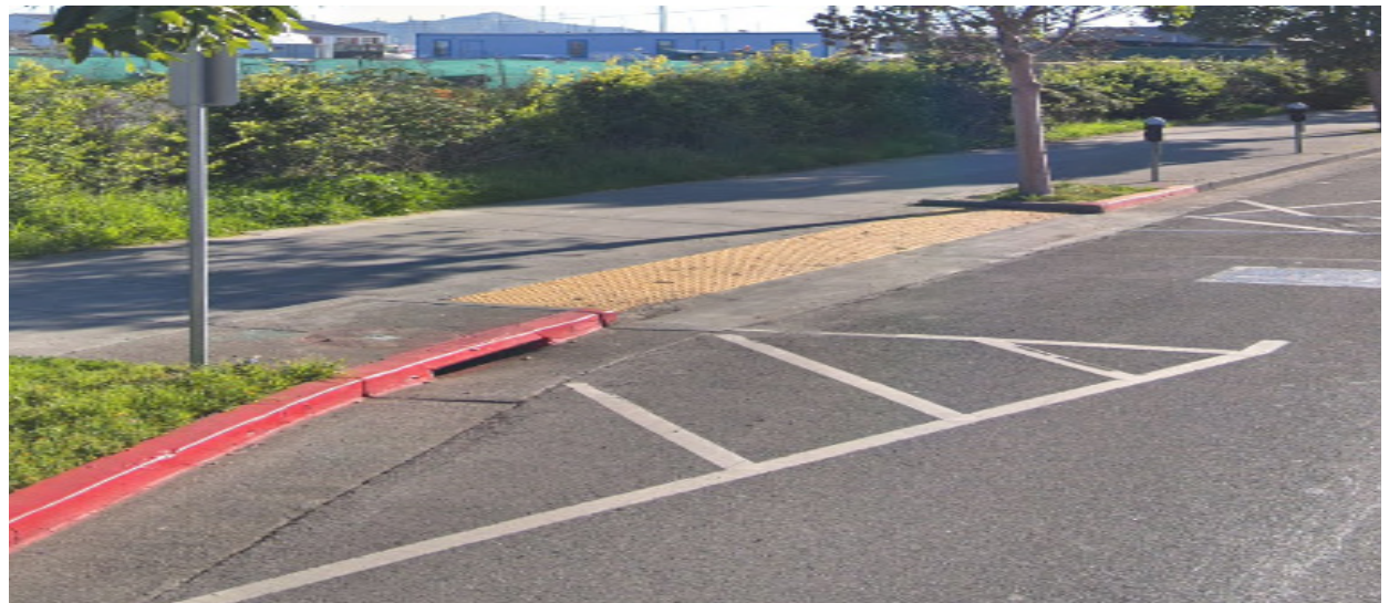
Mid-block curb ramp
