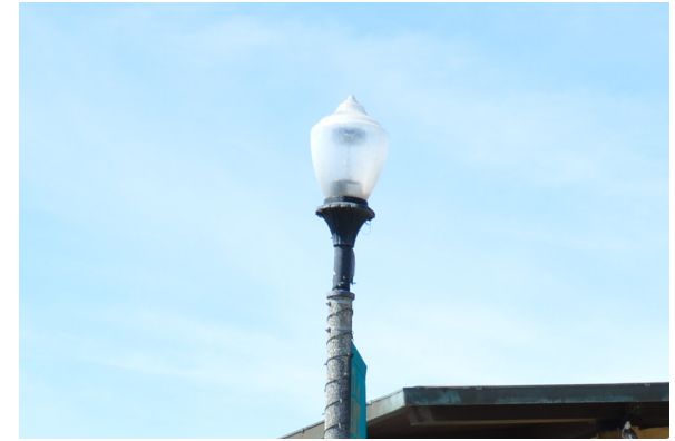
Existing Light Poles
