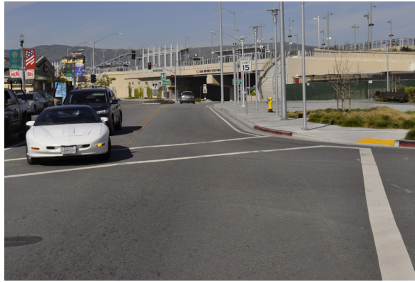
Newly replaced asphalt
