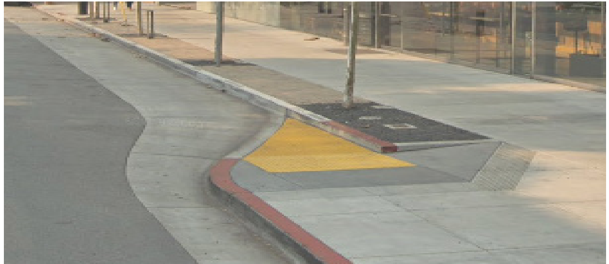
Curb ramp at bulb-out
