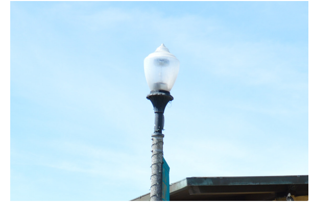
Existing Light Poles
