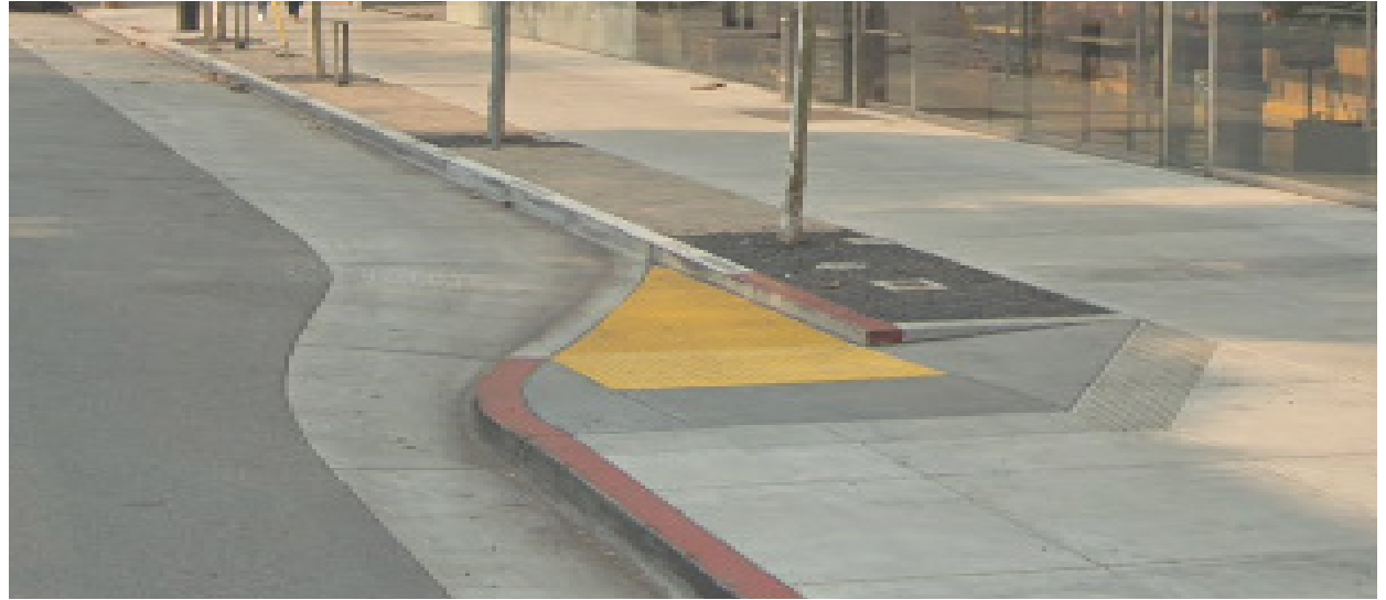
Curb ramp at bulb-out
