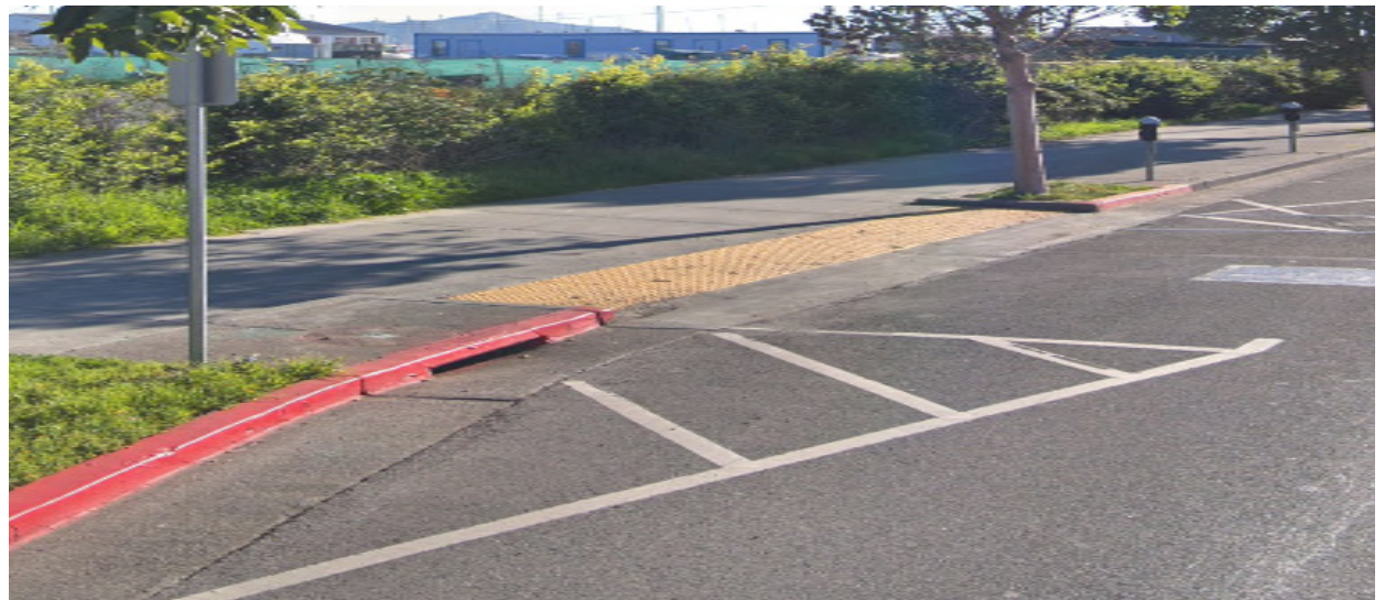
Mid-block curb ramp
