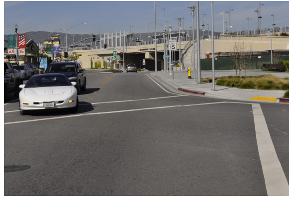
Newly replaced asphalt
