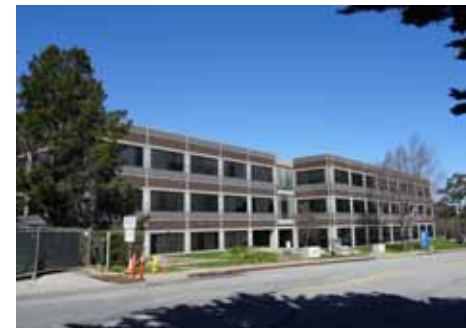
The design of this three-story office building on Grundy Lane emphasizes the horizontal. It incorporates a variety of colors and textures but exhibits minimal facade articulation.
