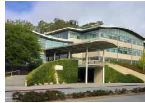
The Gap-owned building leased by YouTube at 901 Cherry Avenue is a contemporary structure that features curved, green rooftops, terraced landscaping, and podium parking. Behind it is the only parking structure in the Planning Area.
