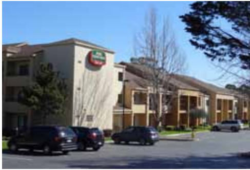
The Courtyard by Marriott San Francisco Airport located at Bayhill Drive and Elm Avenue is a typical two-story auto-oriented hotel with surface parking on three sides.
