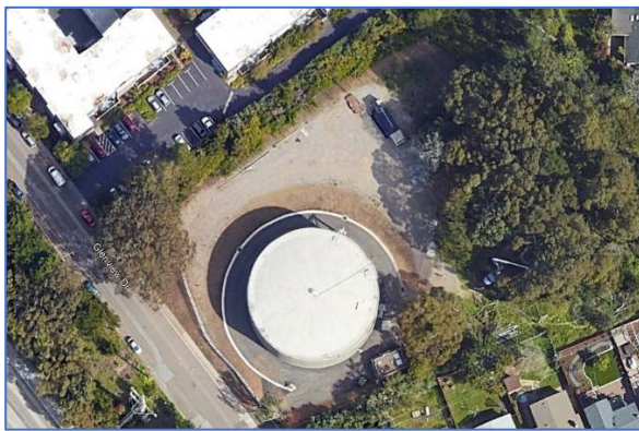
Google Earth Imagery – Water Storage Facility
