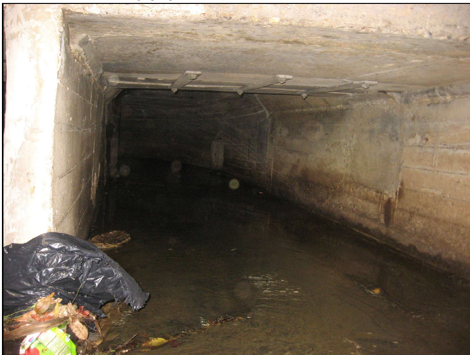
Downstream Channel (right)
