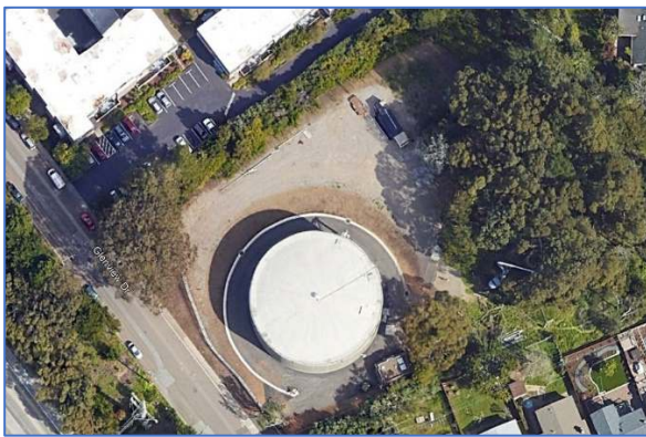
Google Earth Imagery – Water Storage Facility
