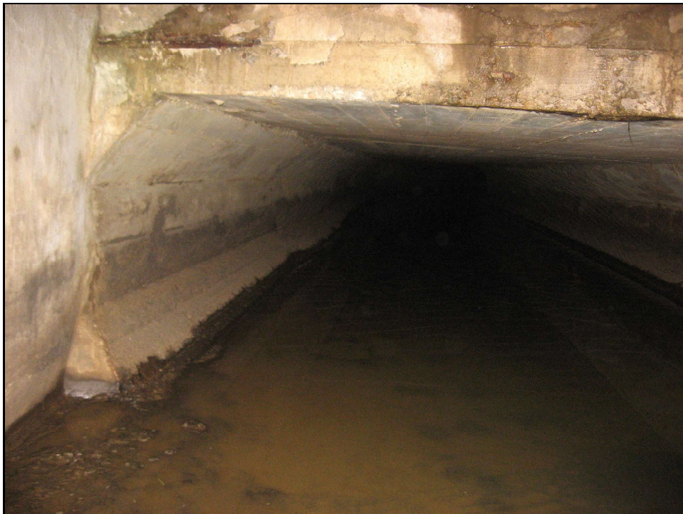
View Looking Upstream
