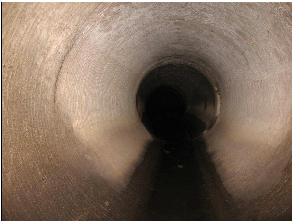
View Looking Upstream
