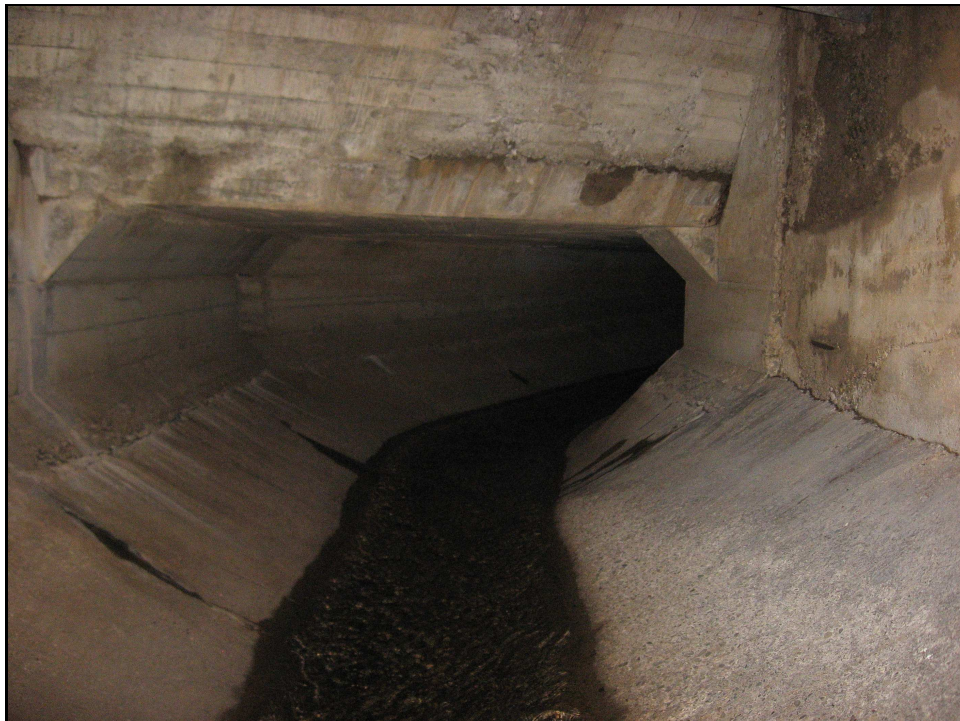
View Looking Upstream
