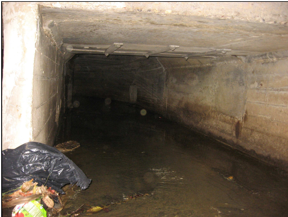
Downstream Channel (right)
