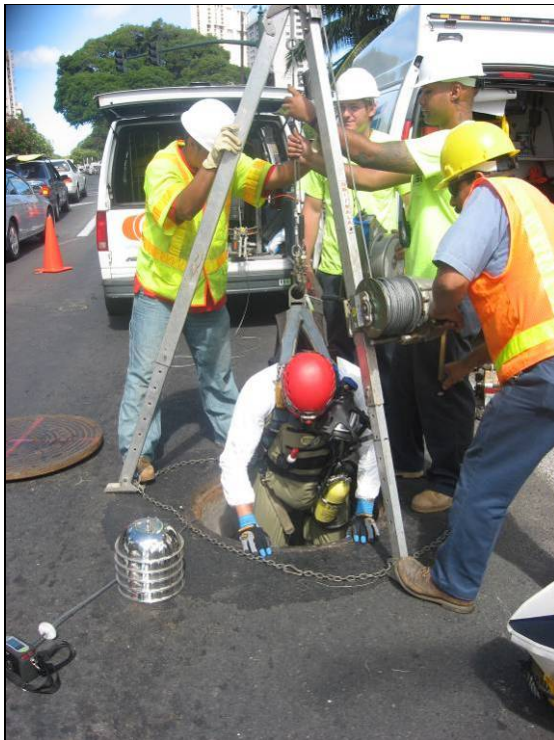
Photo 1. Confined Space Entry
