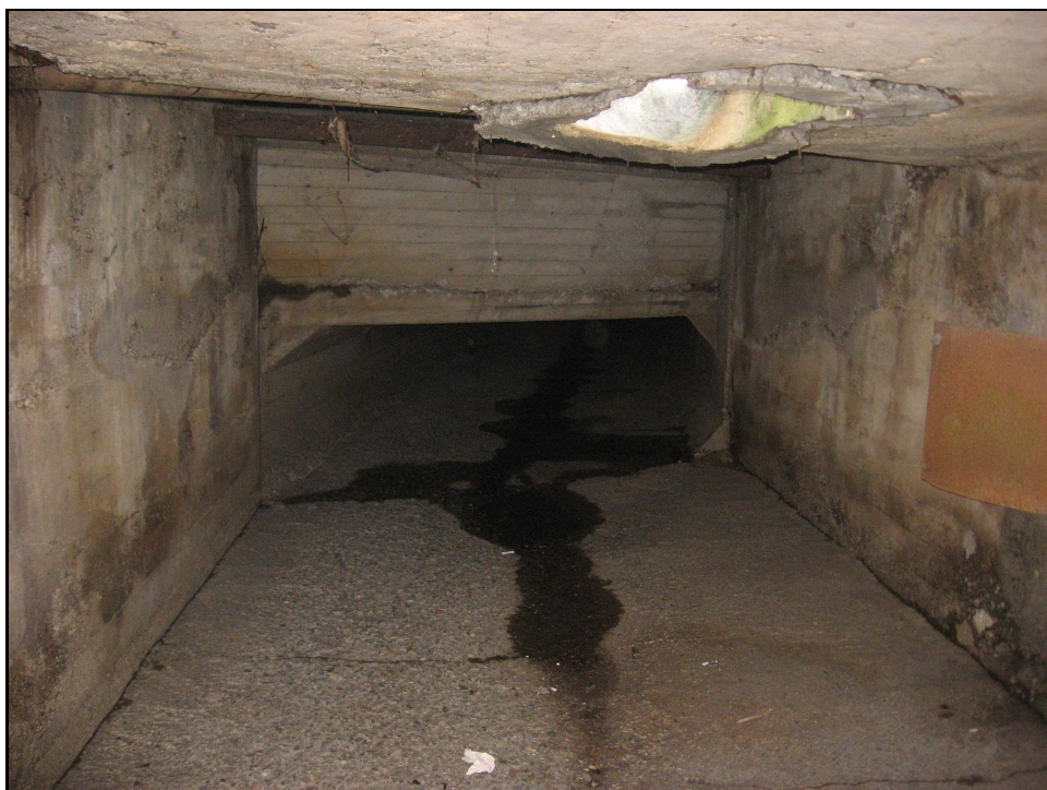
Downstream Overflow Channel
