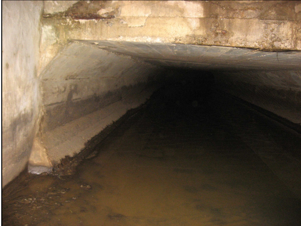
View Looking Upstream
